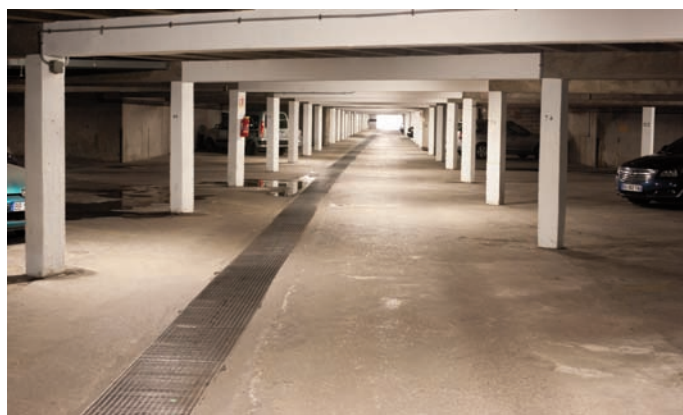
Parking souterrain de Zilina
